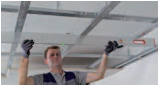
Align the CD-profiles using a spirit level or laser level.
