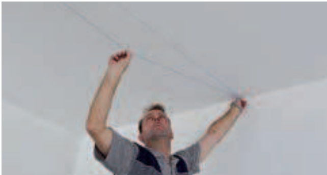
Mark out the ceiling module from the centre of the room, for example using a chalk line. Ensure the margins at the sides of the room are identical.
