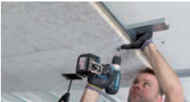
Install the acoustic tiles with the aid of a support. When fixing, press the tile onto the profile using the heel of your hand. There must be no gap between the tile and the profile. Begin tile installation from the centre of the room. Only handle the acoustic tiles with clean hands (clean gloves are recommended) and clean tools.
