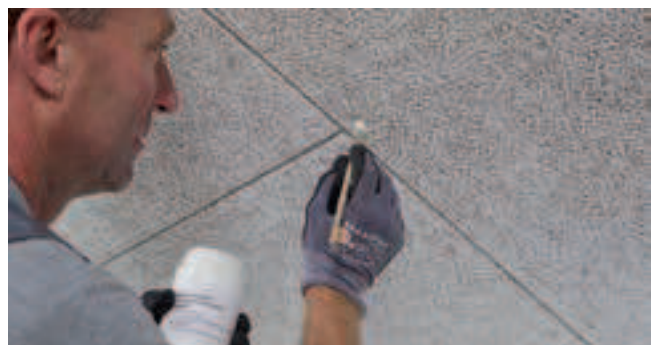
If coloured screws are not used, paint over the screw heads with the paint supplied or a suitable equivalent using a fine brush and suitable amount of paint. Screw heads must be flush with the tile surface.
