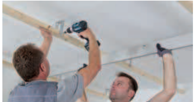
Align the battens using a spirit level or laser level and fix the battens to the hangers, e.g. quick hangers, using 2 screws per side.
