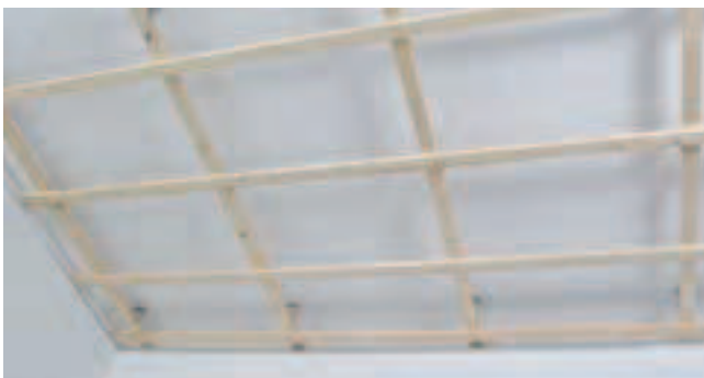
Install the primary and main battens. Maximum centres according to the “Maximum centres of the substructure” table for screw-fixing onto wooden battens and the primary/main batten connection detail.
