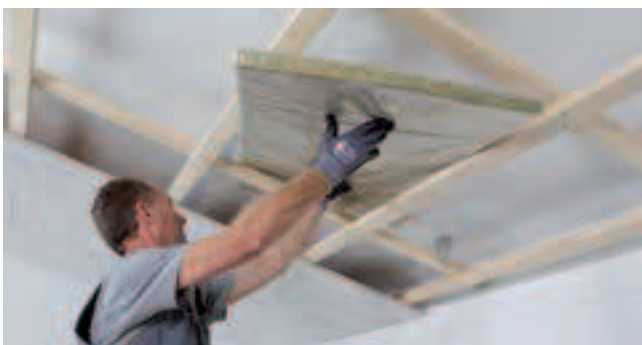
Insert HERADESIGN® acoustic overlays or other acoustic overlays, step-by-step when installing the HERADESIGN® acoustic tiles. Absorber tiles that are pushed between the wooden battens are cut to size.
