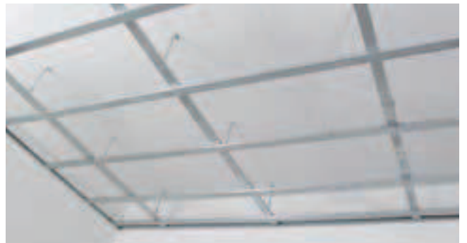
Finished ceiling grid.
