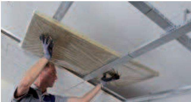
Insert HERADESIGN® acoustic overlays or other acoustic overlays, step-by-step when installing the HERADESIGN® acoustic tiles. Absorber tiles that are pushed between the CD-profiles are cut to size.
