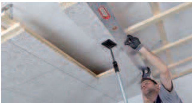
Align the rows of tiles with an installation batten. Tile joints must be positioned centrally under the battens. No free tile joints are allowed.
