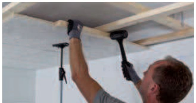
Close possible gaps between the tiles using a wooden block and hammer. Only handle the acoustic tiles with clean hands (clean gloves are recommended) and clean tools.
